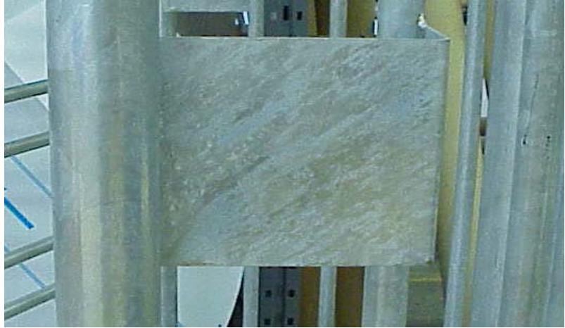
Fig.18 Mounting plate for access control devices
